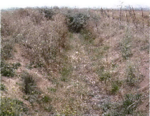
Figure A4. Central drainage on project site.
