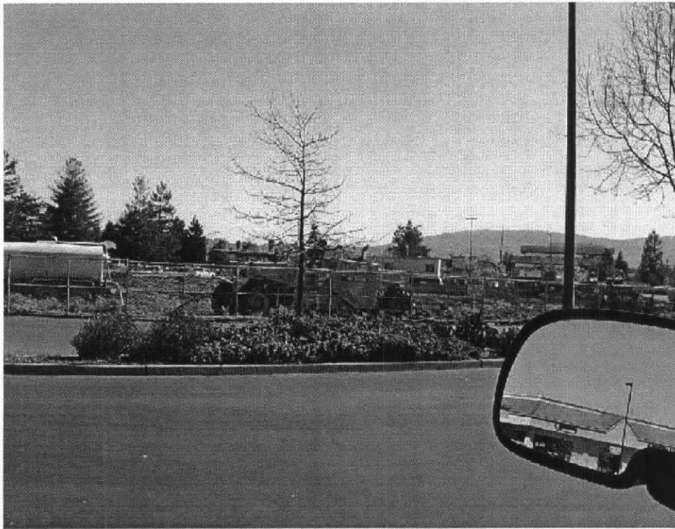
Looking east at construction at 321 Rohnert Park Expressway
