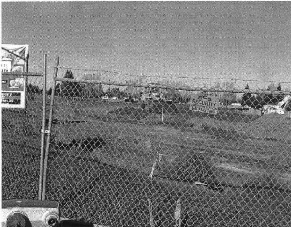
Looking west at construction at former PG&E Facility (600 Rohnert Park Expressway)
