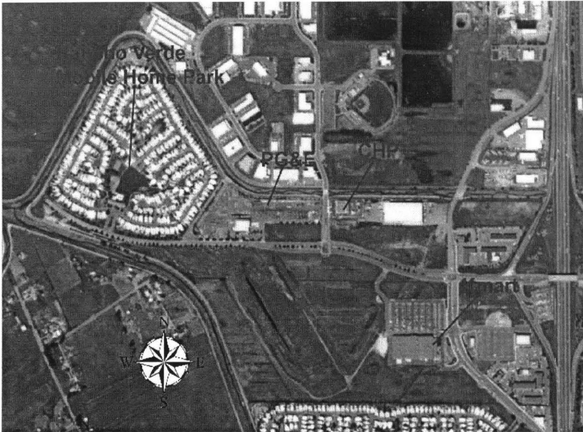
Aerial Photograph Dated March 1987 In this photograph, additional development has taken place. The photo shows that the PG&E building is on the former Site. A K-Mart store has been constructed; additional hotels and a mini mall have been constructed as well. Very few traces of the Former NAAS OLF Cotati facilities are visible.
