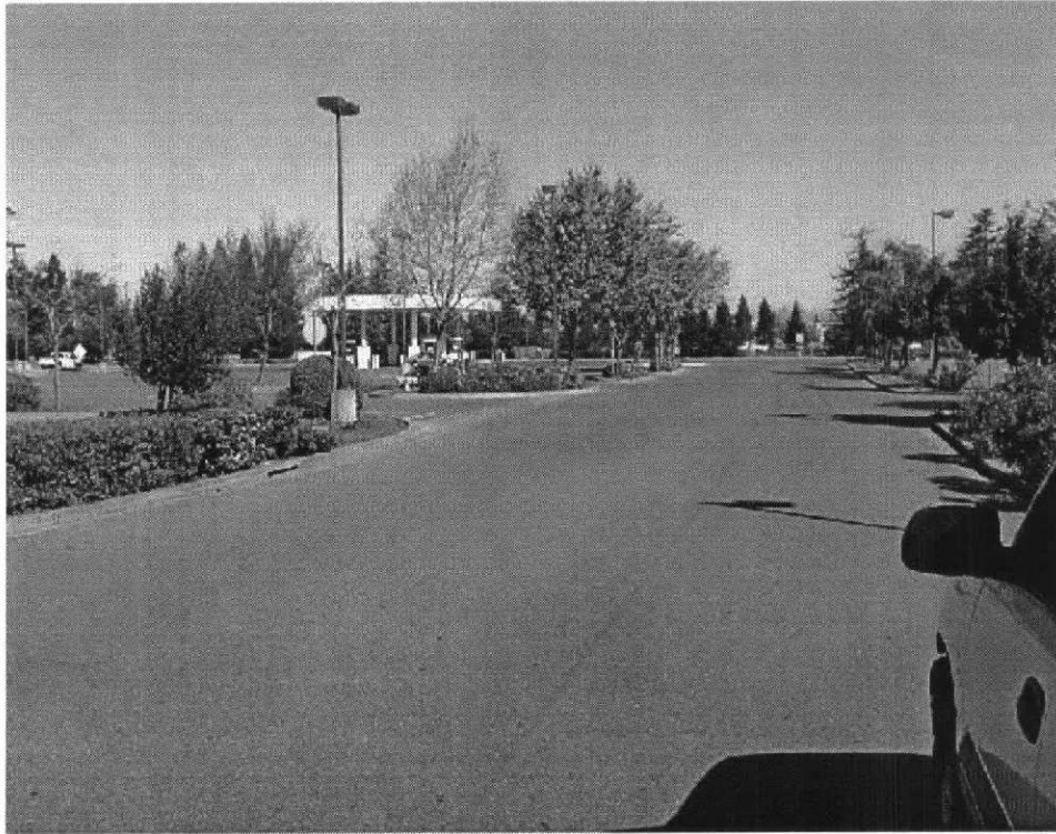
Looking north at a gas station at 561 Rohnert Park Expressway
