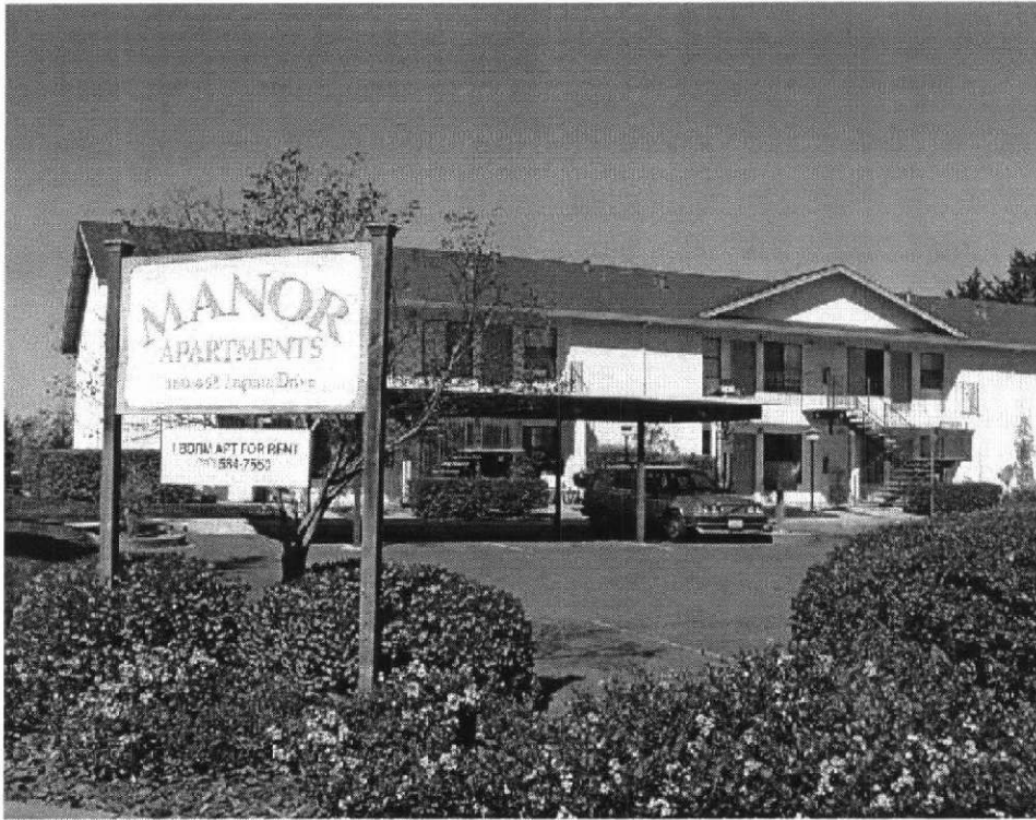
Looking west at Manor Apartments (360-458 Laguna Dr)
