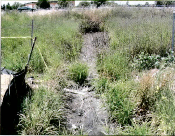
PHOTO 21 At the southwest corner of Intersection #9 looking west
