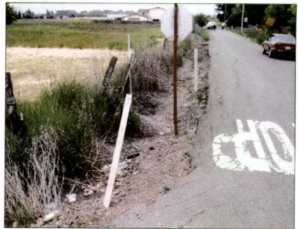
PHOTO 16 At the southeast corner of Intersection #6 looking south
