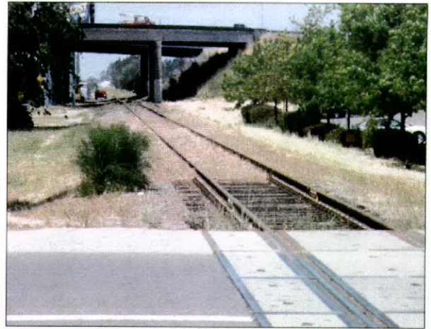
PHOTO 22 At the southwest corner of Intersection #10 looking north
