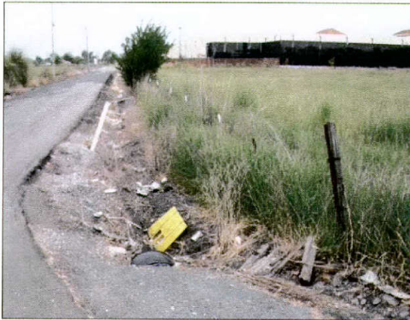
PHOTO 15 At the northeast corner of Intersection #6 looking north
