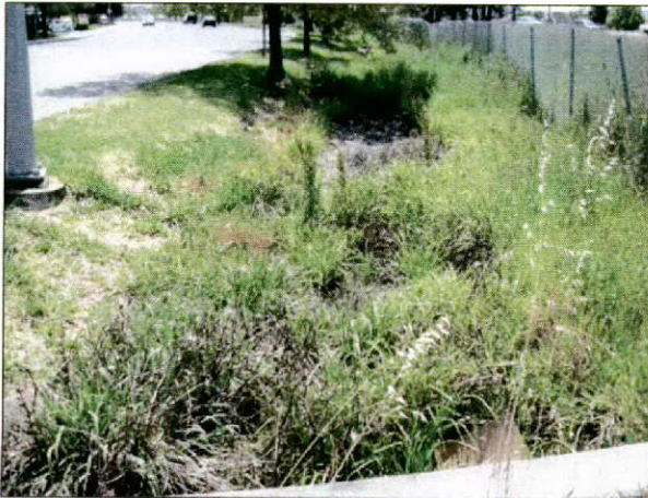
PHOTO 25 At the southwest corner of Intersection #11 looking south
